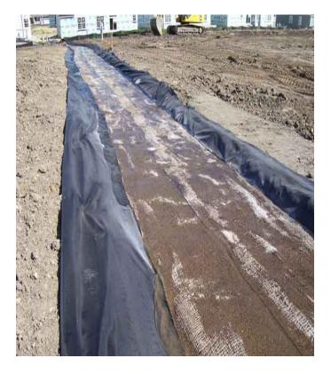
By the time the water flowed down the entire channel, the water was well within discharge clarity requirements, and with no aquatic toxicity potential, could be directed into the storm drain system with no further treatment.
